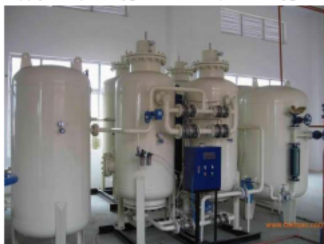
Image 3 : PSA oxygen plant
